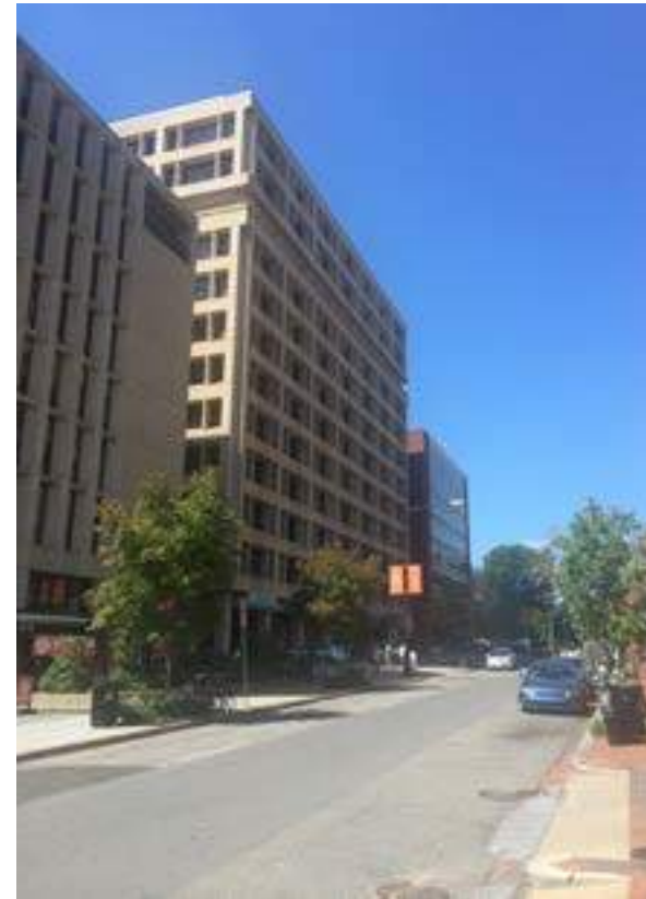
2. 19th Street from South
