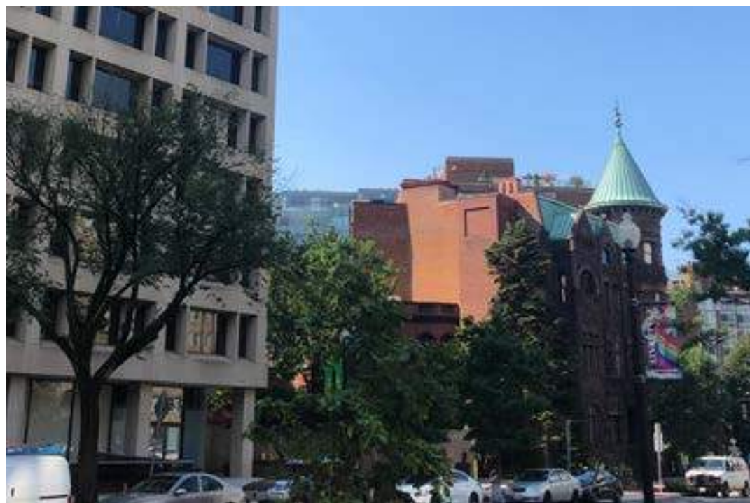
4. Heurich House from North
