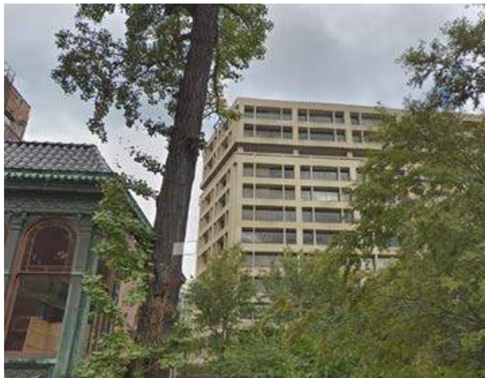
2. South Facade from Heurich Property
