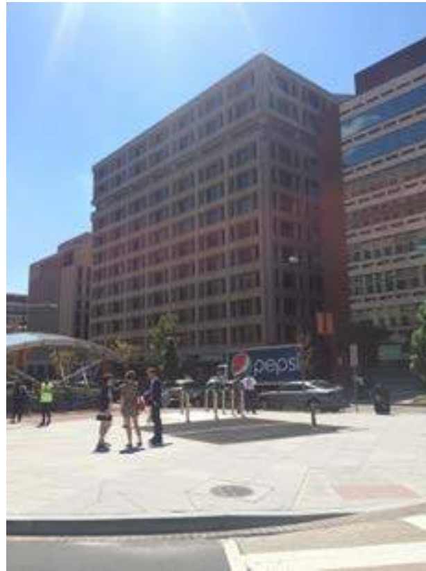
1. 19th Street from North
