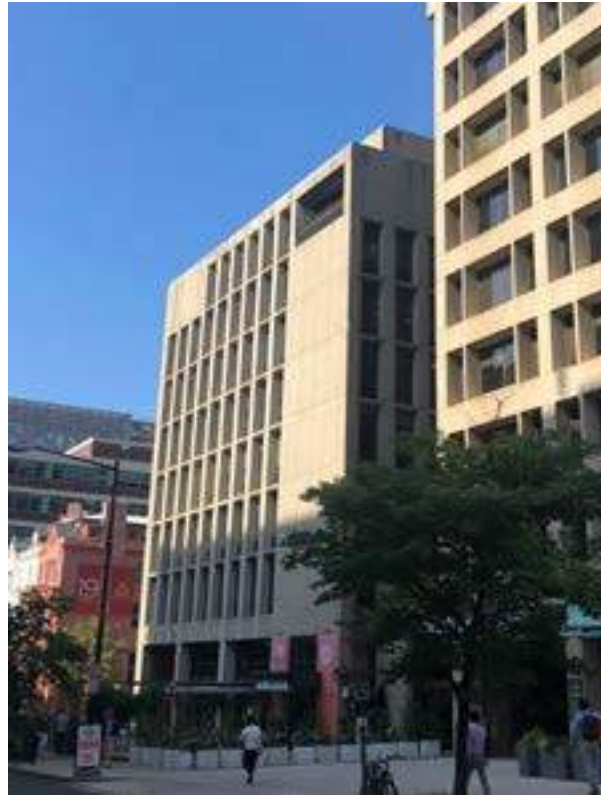
3. 1320 19th St NW From North
